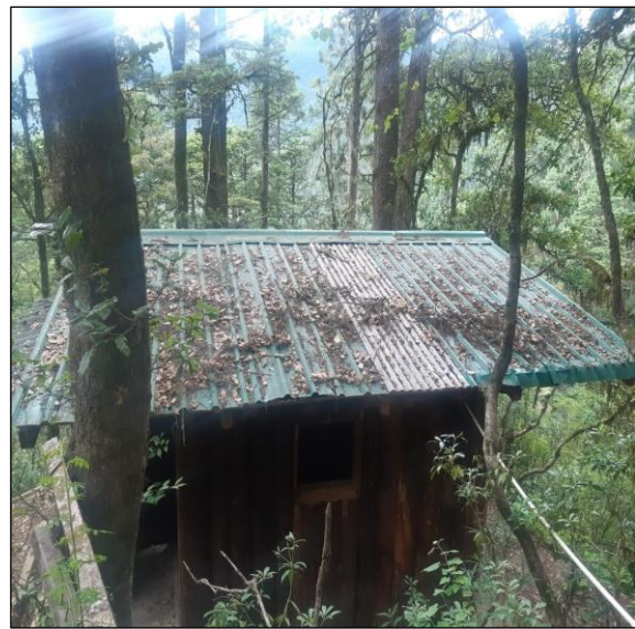
Figure: Restroom two
