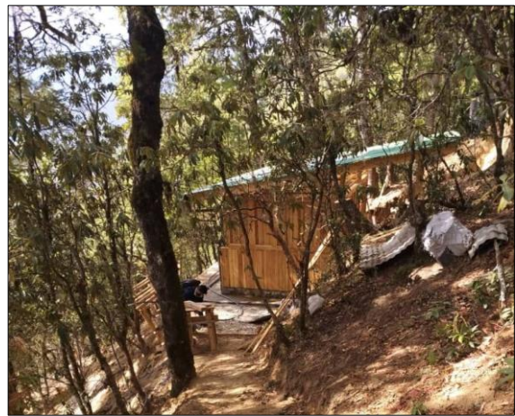
Figure: Restroom two
